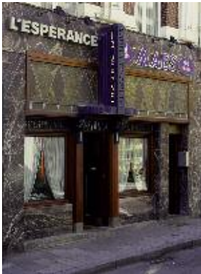
Taverne L'Espérance, Finisterrastraat 1-3 in Brussel. Architect Léon Govaerts, 1930.
