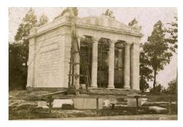
The Pavilion of Human Passions, arch. Victor Horta, before 1893. View during construction. The relief is not yet in place (note the brick wall at the back) and the capitals have yet to be carved. The building is still without a roof.
