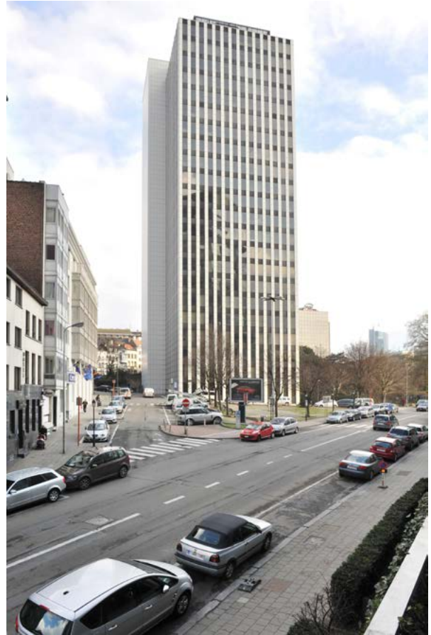
AFB. 1B Victoria Tower in 2022 (T. Verhofstadt © urban.brussels).
