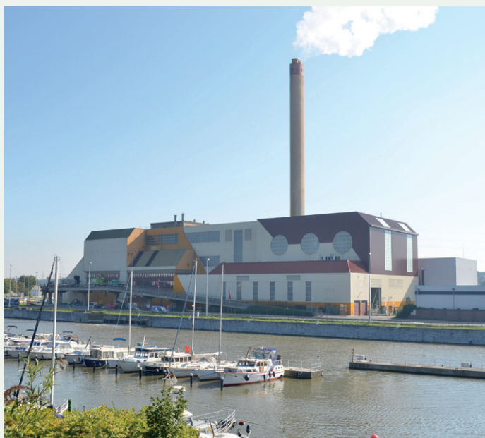
Afvalverbrandingsoven (© Brussel Energie SCRL).
