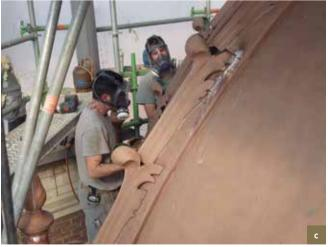
Le Roi d'Espagne/Den Coninck van Spaignien. Stages in the restoration of the copper cupola. a) Condition of cupola before restoration with dirt and green patina; b) and c) Sandblasting in progress to expose and restore the copper in order to replace damaged parts and repair defective welding, among other things d) Cleaning and polishing using steel wool (© HHU, 2015).
