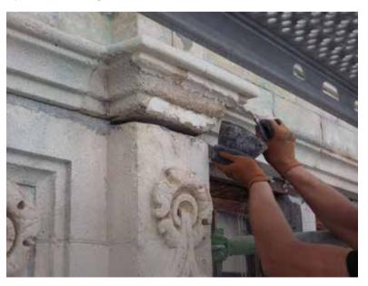
${\it La~Brouette/Den~Cruywagen.}~{\it Mouldings~undergoing~restoration~and~repair~with~smoothing~mortar.~Euville~stone~(©~HHU, 2014).}$
