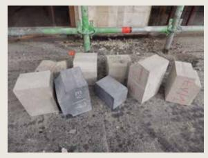
New stones delivered to the worksite to carry out the repairs required as a result of the chipping of stones due to corroding metal elements. Gobertange stone and blue stone (© HHU, 2015).
