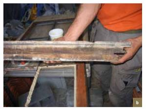
La Rose/De Roose. Damaged oak wood pieces. a) A weatherboard (lower part of window frame) requiring replacement; b) A window sill requiring replacement (© HHU, 2014).
