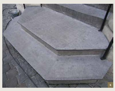
Le Cygne/De Swane. a) Chiselling of entrance steps in progress, based on the existing model. Blue stone; b) Finished job (© HHU, 2008).
