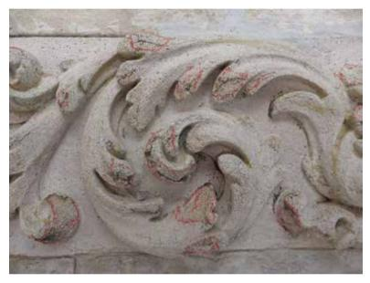
La Brouette/Den Cruywagen. Detail of scrollwork with red chalk marking the parts to be repaired with smoothing mortar. Euville stone [© HHU, 2014].
