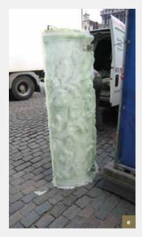
La Maison des Brasseurs/Het Brouwerhuis. Column decorated with twisted foliage. a) The metal parts caused the element to crack or chip (cementing on original stone). Damaged state before casting and restoration; b) Core sampling of mortar; c) Moulding with silicone; d) Fibreglass-reinforced polyester resin shell; e) The cast is transported for possible reproduction; f) Finally, the elements were restored *in situ*, painted and gilded (© HHU, 2014-2015).
