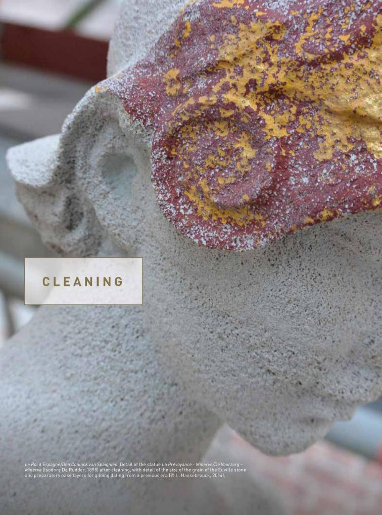
The purpose of the cleaning process was to remove all forms of dirt and deposits on the facing. This operation had to ensure that the calcin layer, which provides natural protection for the stone and gives it its patina, was preserved.
