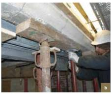
Sainte-Barbe/Sint Barbara. a) Detail of the stone to be replaced, marked with a cross using red chalk; b) New Gobertange stone elements and stainless steel bars (© HHU, 2015).
