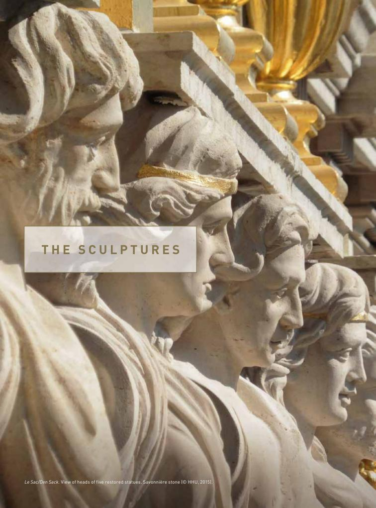
The Grand Place has a rich collection of sculpted ornamentation. This element has undergone light restoration using repair mortar. In rare cases, where the details had become unrecognisable or the piece was deemed to be too badly damaged, it was replaced, provided that complete, reliable information (old archives, photographs) was available. Mouldings were then taken of the existing sculptures beforehand.
