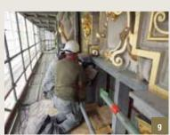
Le Sac/Den Sack. Stages in restoring a capital: a) Damaged condition; b) Removal of element; c) Moulding of a capital in good condition; d) Silicone mould with fibreglass-reinforced polyester shell; e) Plaster positive; f) New sculpture made from Savonnière stone; g) Integration of the stone element [© HHU, 2014-2015].
