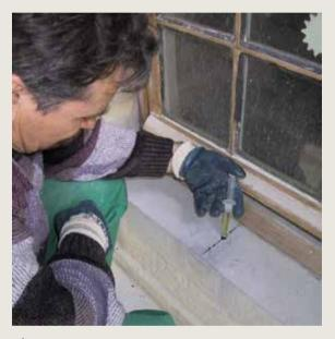
$L'\hat{A}$ ne/Den Ezel. Blue stone threshold. Injection of product [two-component epoxy] via small holes prepared for this purpose [© HHU, 2003-2004].
