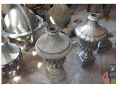
Le Sac/Den Sack. Zinc vase. a) Cracked and pockmarked original element; b) Old and new elements (© HHU, 2014-2015).
