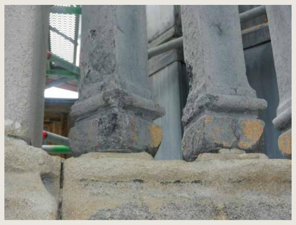
*Le Roi d'Espagne/Den Coninck van Spaignien.* Pitting of the stone due to the presence of stylolites and the face-bedding of the stone in the balusters. Blue stone (© HHU, 2014).
