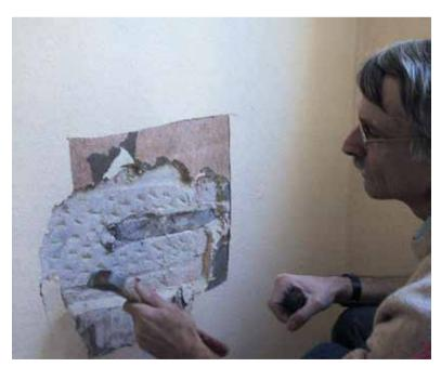
$L'\hat{A}ne/Den$  Ezel. A. Pien removing the render from a party wall to determine the shape of an anchor (© CHE, 2001).
