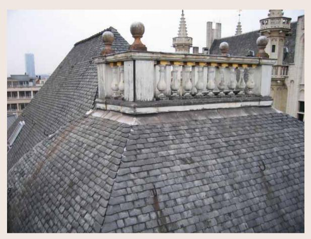
*Le Cygne/De Swane*. Wooden terrace on belvedere. Dislocated elements. Lower sections damaged. Widespread lack of maintenance (© HHU, 2008).
