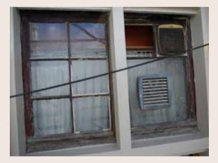
La Chaloupe d'Or/De Gulden Boot. Two window frames with damaged weatherboards and window sills. The frames were modified over time to incorporate ventilation outlets in a random fashion (O HHU, 2014).
