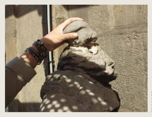
Le Renard/De Vos. Powdering of an Euville stone sculpted feature, causing the rupture of an element (© HHU, 2014).
