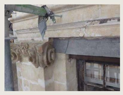
Le Pigeon/De Duive. Crack in the blue stone lintel caused by the development of rust on the metal lintel ( HHU, 2012).
