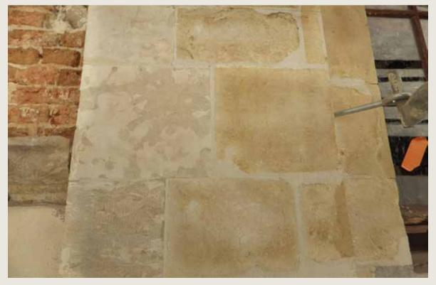
Le Heaume/Den Helm and Le Paon/Den Pauw. Detail of facing after cleaning showing the Gobertange stone facing (on the left) and the Balegem stone facing (on the right) on the façade of Le Heaume/Den Helm. The brick masonry on the façade of Le Paon/Den Pauw can be seen on the far left of the photo. This was revealed after the removal of loose render (© HHU, 2015).
