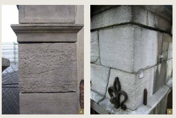
L'Étoile/De Sterre. a and b) Separation and open joints in the Euville stone as a result of structural problems (pressure from corroded metal elements in the floor) (© HHU, 2008).
