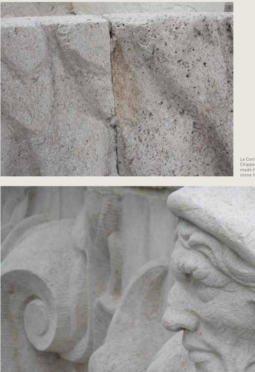
*Le Cornet/Den Horen.* Chipped element made from Euville stone (© HHU, 2014).
