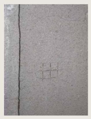
La Chaloupe d'Or/De Gulden Boot. Cement render with wire mesh reinforcement appearing on the surface with presence of rust (© HHU, 2008).
