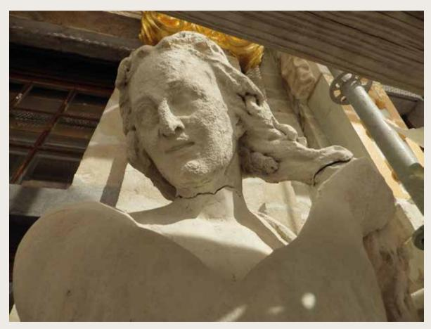
La Louve/De Wolvin. Statue with broken head (due to the corrosion of a dowel pin) (© HHU, 2014).
