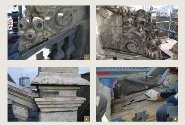
La Chaloupe d'Or/De Gulden Boot. a) Left side aileron with flower motifs. The element is becoming detached and sliding outwards as a result of a corroding metal pin; b) Idem. Right section. Installation of temporary protective net following the inspection, while awaiting the restoration work; c) Displacement of right pinnacle of gable; d) Idem on left side. Beneath the lead, rust can be seen on the metal pin causing the aforementioned problems (© HHU, 2000).
