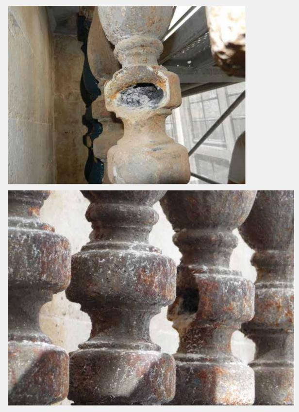
Le Sac/Den Sack. Corrosion of metal balusters, leading in some cases to the total degradation of material (© HHU, 2014).
