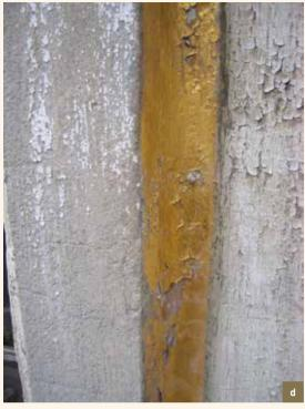
La Chaloupe d'Or/De Gulden Boot. a) Detail of pediment. Flaking paint and gilding; b) An angel. Build-up of dirt on paint. Gilding missing; c) Detail of inscriptions on the tympanum. Cracked render. Paint missing. Damaged gilding; d) Detail of pedestal of pilaster with flaking paint and gilding (© HHU, 2012).
