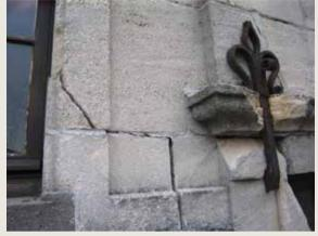
Le Cerf/De Heert. Cracks in a blue stone due to the rusting of the metal ring ( $\textcircled{\mbox{\scriptsize o}}$  HHU, 2000).
