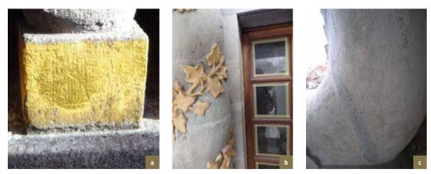
Stone markings. a) *L'Âne/Den Ezel.* Marking on a cube of blue stone; b) *La Brouette/Den Cruywagen.* Numbered stones. Balegem stone; c) *La Maison des Brasseurs/Het Brouwerhuis.* Marking at the back end of a blue stone sculpted dolphin (© HHU, 2002 et 2014).
