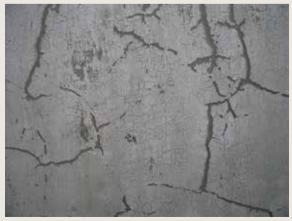
Le Mont Thabor/Den Bergh Thabor. Side façade. Cracking of the render and flaking of the paint ( $\odot$  HHU, 2014).
