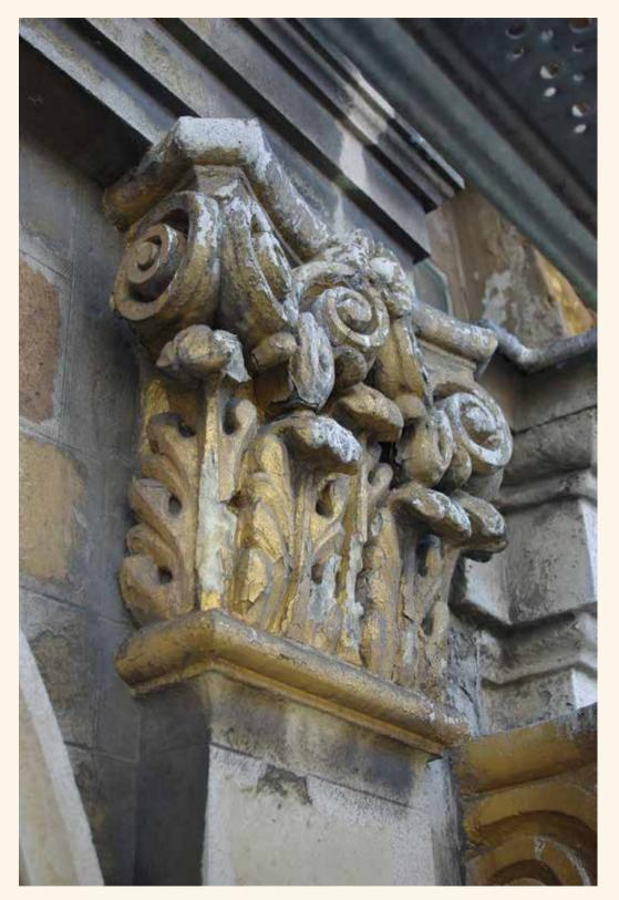
Le Pigeon/De Duive. Detail of a composite capital. Chipping of stone leading to damage to the gilding. General wear and tear of the gilding, build up of dirt (© HHU, 2012).
