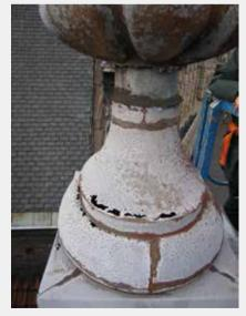
*La Rose/De Roose.* Detail of a corroded and pockmarked zinc vase (© HHU, 2000).
