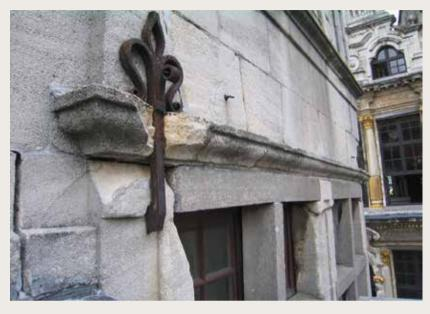
Le Cerf/De Heert. Euville stone exhibiting fracture caused by the corrosion of a metal anchor (© HHU, 2000).
