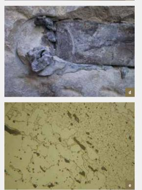
L'Âne/Den Ezel. Metal anchor. a) Locating anchors by means of a metal detector; b) Square plate visible on the façade behind the crumbling facing; c) Stripping of interior plaster in order to see the shape of the anchor; d) Detail of lead anchor in the stone: e) Metallographic study. Micrograph image (a, b, c en d) : © HHU. 2001; e] : © VUB, 2001).
