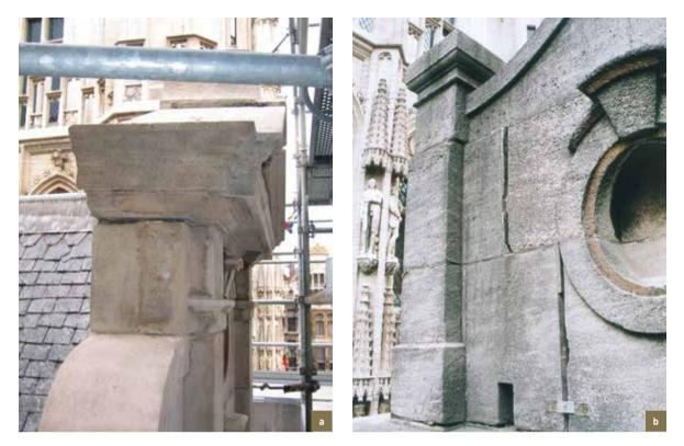
L'Étoile/De Sterre. Structural problems. a) Tilting of gable pediment on the façade facing the Grand Place. Euville stone; b) Separation of stones in the rear façade. Crack meter installed during the schedule of condition (© HHU, 2008).
