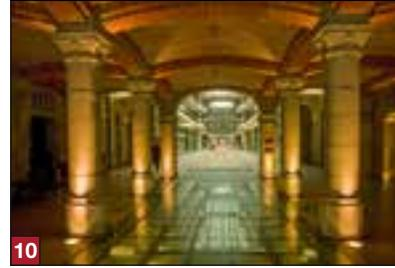
all made from Hennebique reinforced concrete. A metal-structured glass roof provides lighting for the four floors which, today, house shops and offices.
